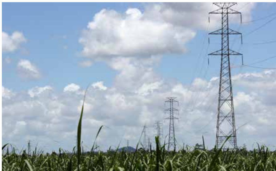
Following years of lobbying from CANEGROWERS and other farm groups, the Queensland Competition Authority confirmed a new electricity tariff which promises to save irrigators money
